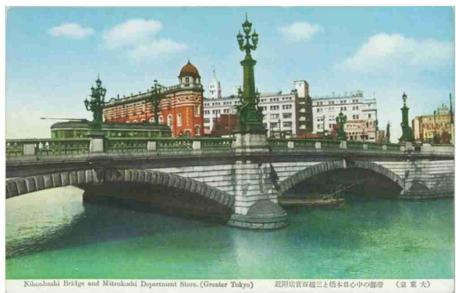
Nishinbashi Bridge and Mitsukoshi Department Store (Greater Tokyo) 近附街貫百越三と橋本日中の都帝 (京東大)
